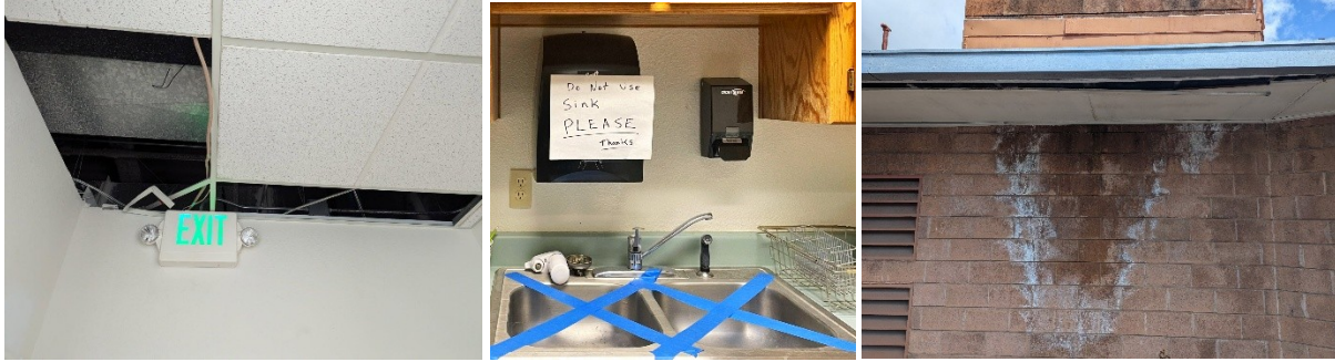
Missing ceiling tiles, unusable facilities, and overhang collapsing due to water damage.
